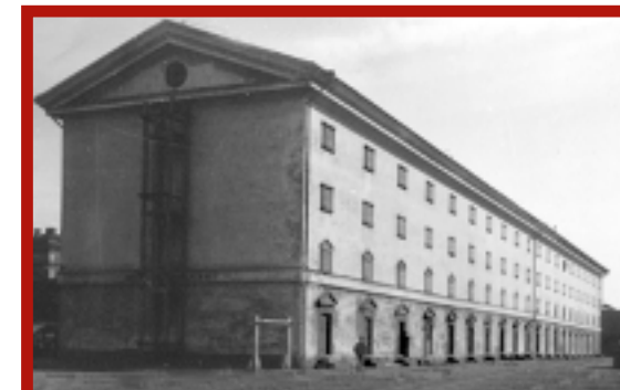
The No. I Storehouse
