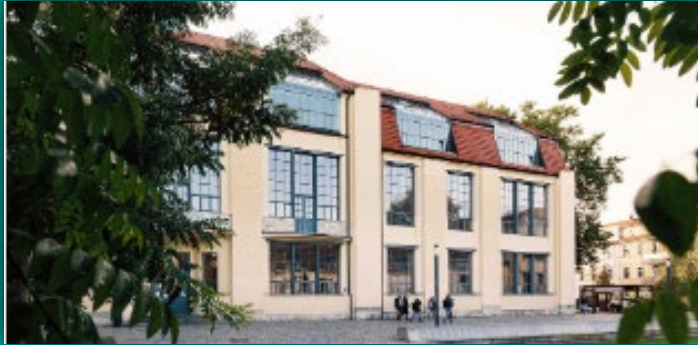
University's main building (primarily used by Faculty of Architecture and Urbanism)
